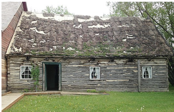
Waldheim House West Wall.
