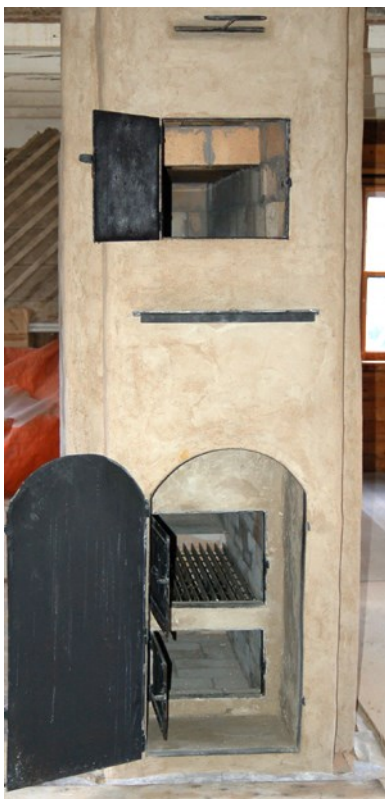
Russian Bake oven- built by masons from restoration Workshop, Parks Canada
