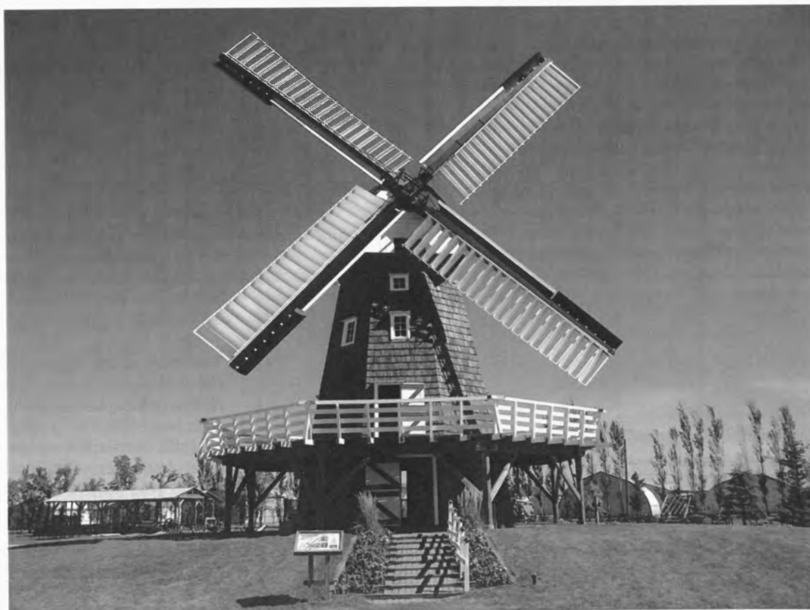
Windmill with its new coat of paint.
