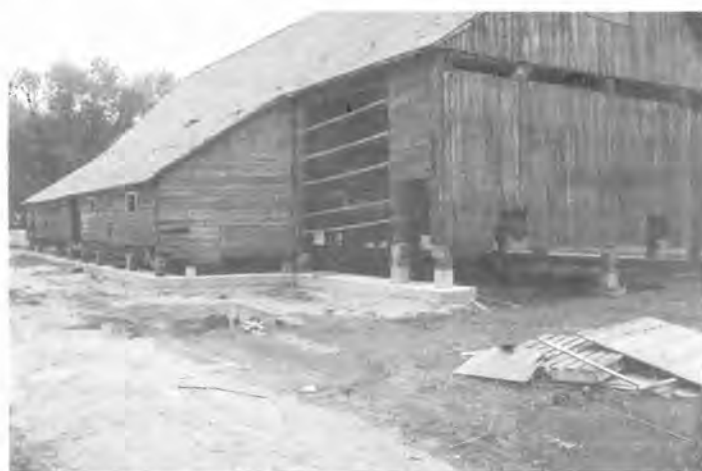
A new foundation was poured for the barn in June 2006. Rotten sills and timbers were replaced with temporary blocks to level and stabilize the structure. Restoration plans are being developed. Photo credit: Jake Peters
